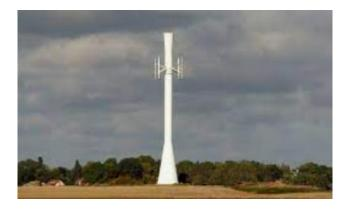
Concrete itself has a lower environmental impact than traditional steel, producing 30% less CO<sub>2</sub> emissions during production and transportation. In addition, the Ericsson Tower Tube does not require feeders and cooling systems. This results in up to 40% lower power consumption than traditional base station sites, helping operators reduce their operating costs significantly.
